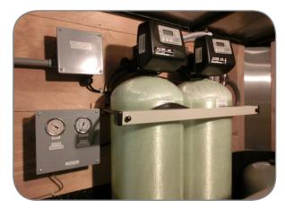
Included with the system, a remote boost pump (all plastic jet pump) with an inlet screen and quick connects on all hoses. Attached inside the trailer are twin tank media filters with automatic back flushing gauges that measure pressure drop across filters
