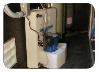
We installed a 125 gallon product water tank with a boost pump. Chlorine is injected into the product water before it enters the product water tank
